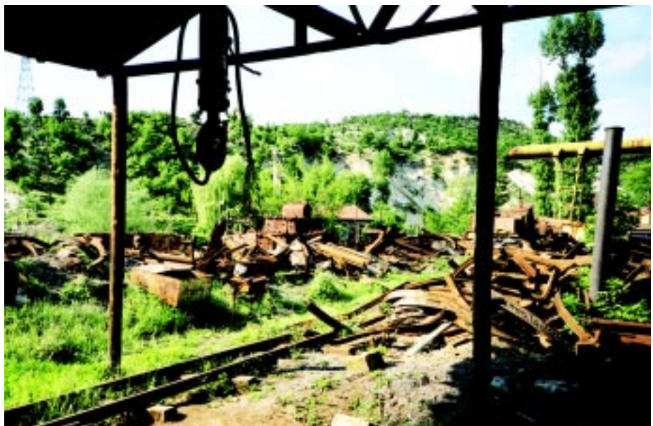
Abandoned surface facilities at the Pirin Mine
