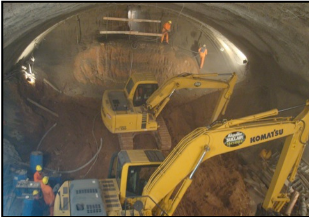
Figure 4. First one-pass lining at garage-workshop in Line A.
