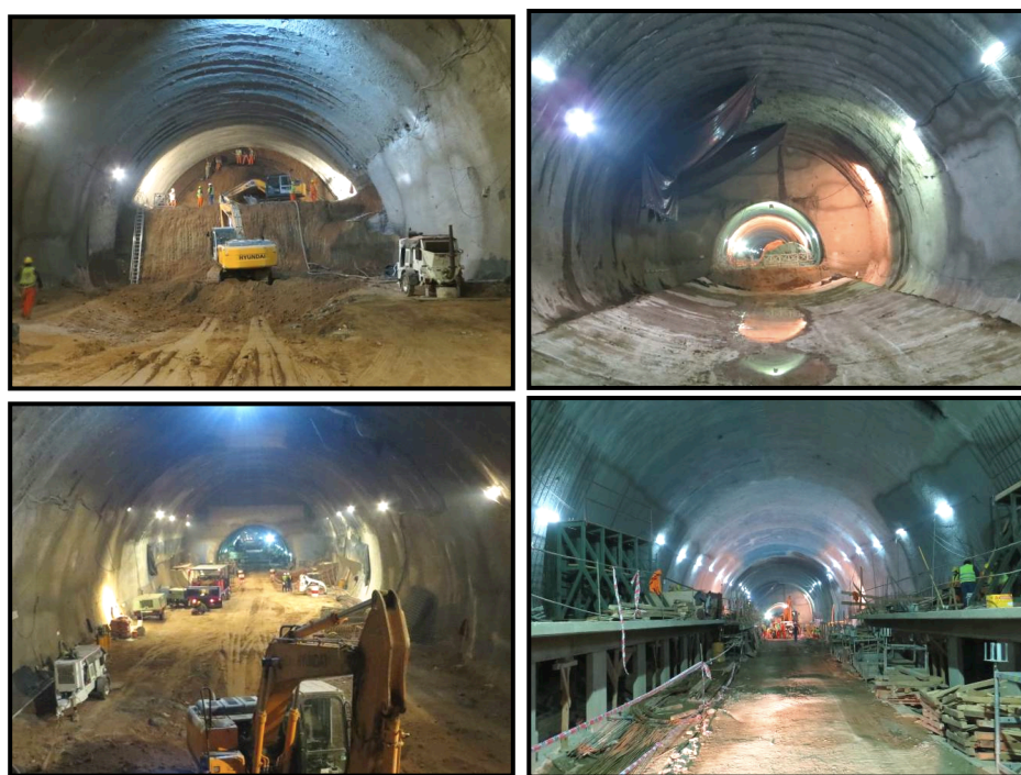
Figure 11. Construction stages of the caverns.
