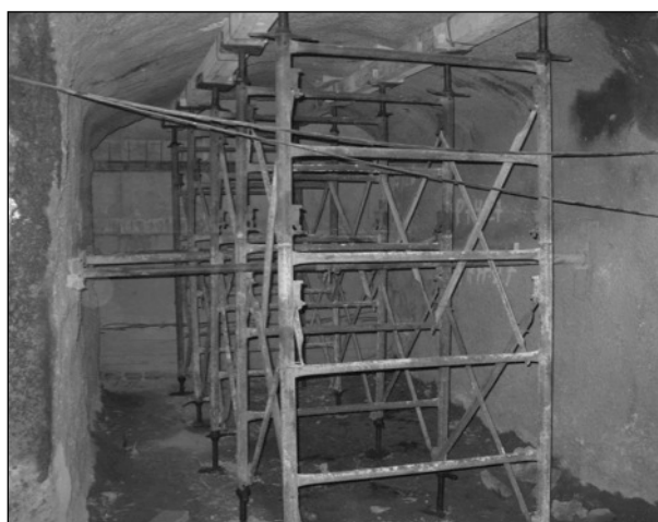
Figure 3. Temporary propping of auxiliary galleries to reduce surface settlements, Echeverria Station.
