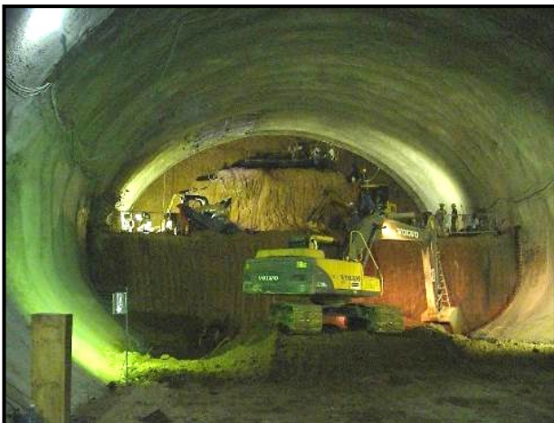
Figure 5. All-shotcrete solution for garage-workshop in Line B.
