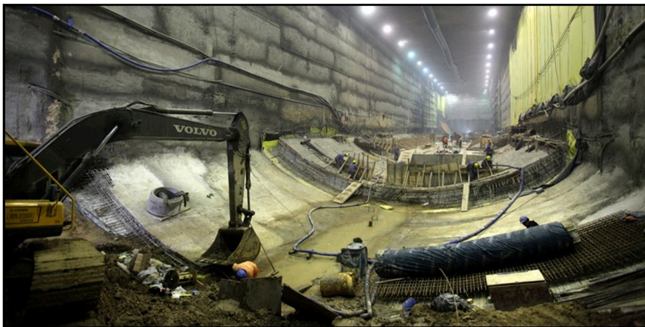
Figure 7. Correo Central station. NATM invert.
