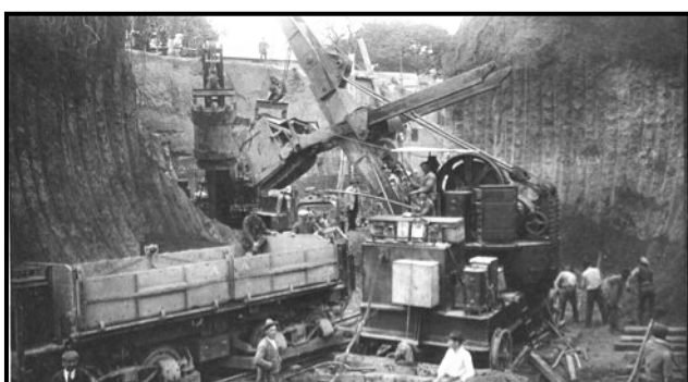
Figure 2. Open pit excavation of Line A in 1912.
