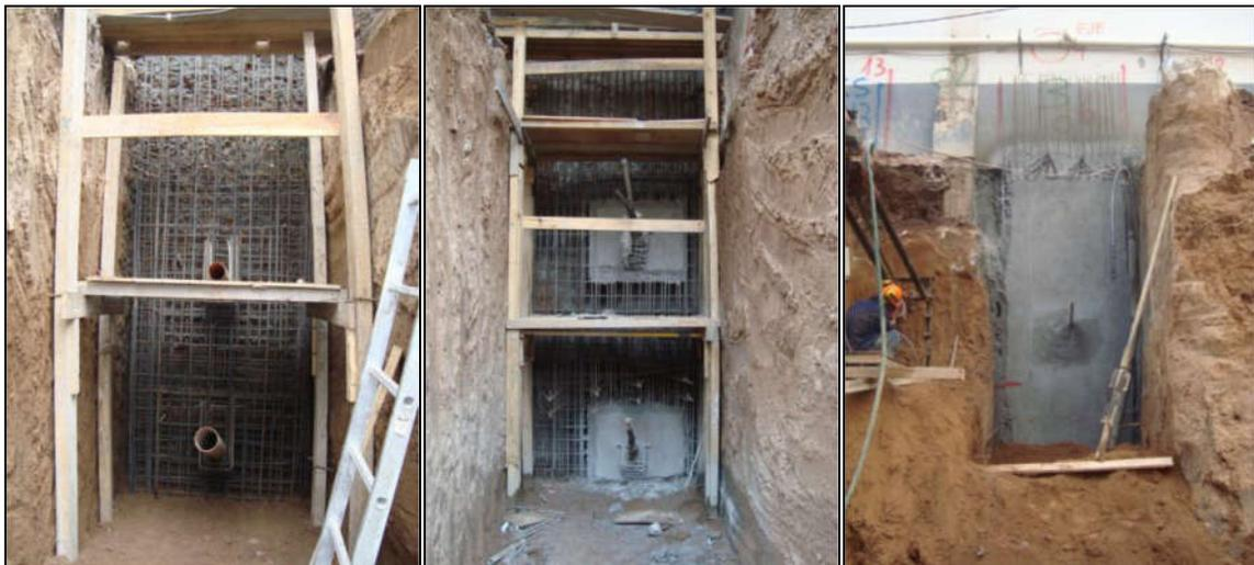
Figure 7. Construction sequence of the anchor plates as part of the final wall (Laríá 2015).
