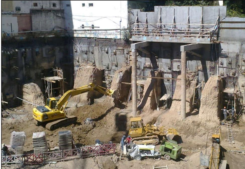
Figure 6. Typical construction procedures for large excavations in Buenos Aires. Real world.
