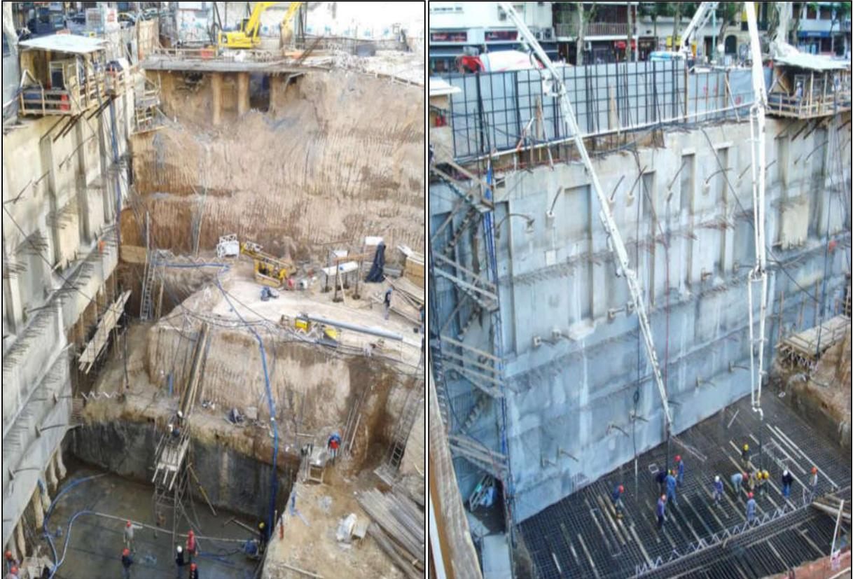
Figure 10. Pile-supported excavation, street side of Vista Tower.
