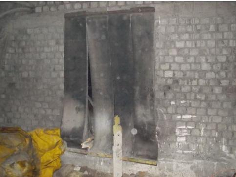
In more and more models that I review, I observe users inputting a resistance value for bulkheads or stoppings that equates to infinite resistance (a total closure of the drift from air).
