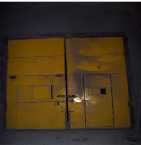
In reality, a zero leakage bulkhead is rarely the case. I have seen this used in a model where the bulkhead with a door actually had 4 m<sup>3</sup>/s leaking through holes. The model had zero leakage. Multiply this by a number of bulkheads in the mine, and your model becomes far less accurate.
