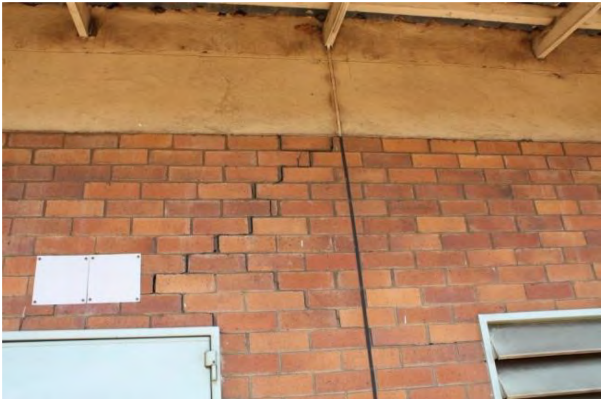
Figure 14-11: Example of blast induced damage
