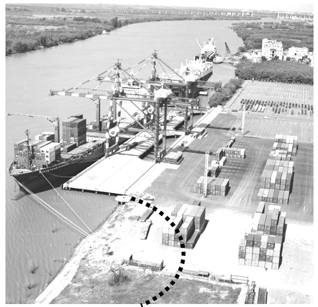
Figure 11. Aerial view of the site after rehabilitation works.
