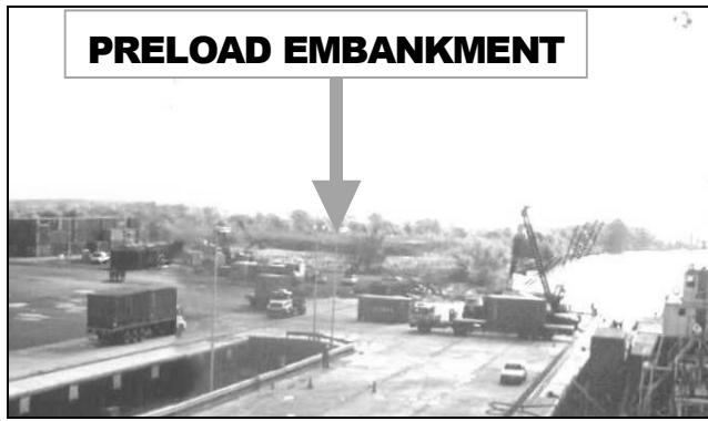
Figure 2. Preload embankment as seen from the wharf.
