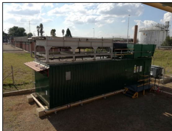
Figure 6-1 (b): Deutz containerised engine
