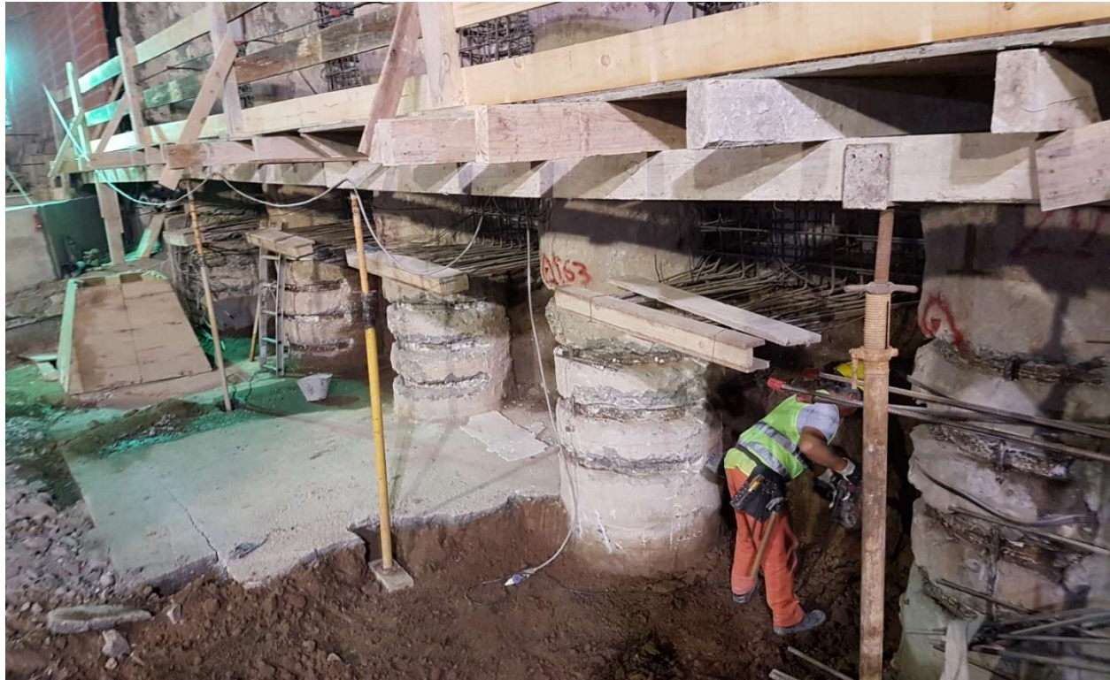
Figure 15. Structural detail of the connection of the invert to the lateral bored piles.
