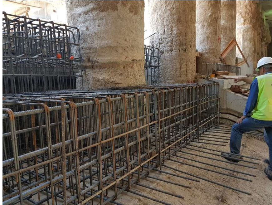
Figure 16. Reinforcement of the slab connected to the (future) wall between the piles.
