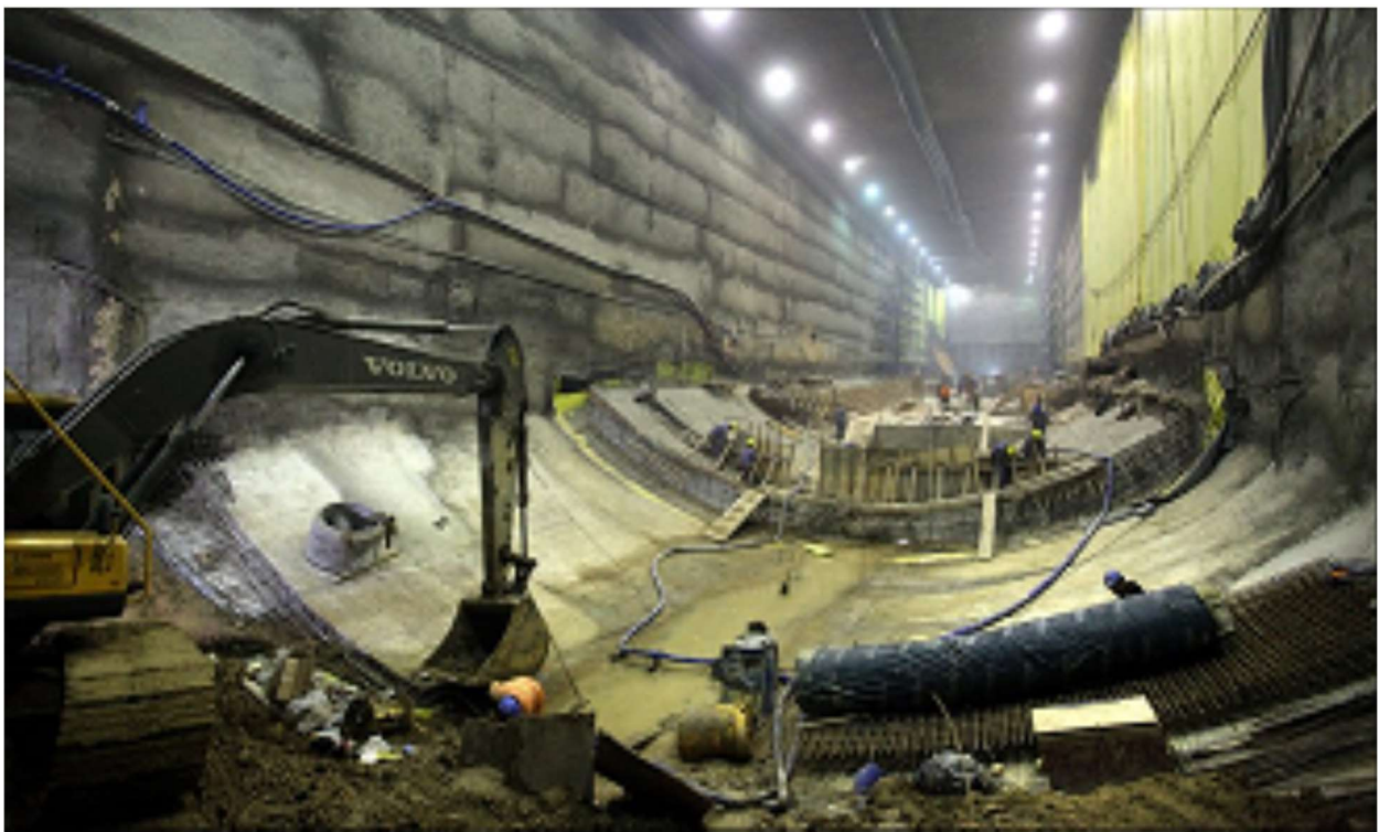
Figure 26. Correo Central Station. All construction stages of the invert including the installation of the geomembrane and the casting of the final invert.
