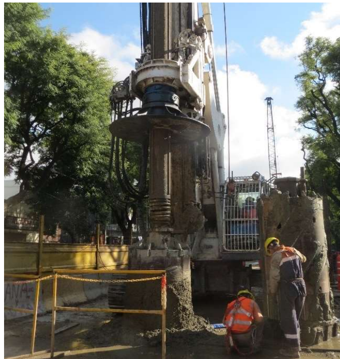
Figure 33. Soilmec SR-70 piling rig provided with two buckets and no casing during the construction of the secant pile wall at Pre-Hospitales tunnel.
