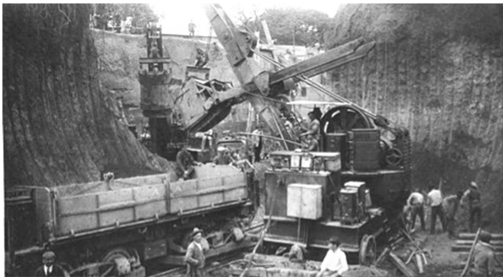
Figure 1. Excavation of Line A in 1911 (SBASE 2017).
