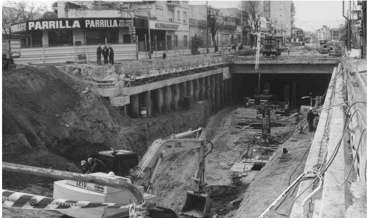
Figure 7. Tronador Station. Note piles with no head support working in cantilever mode.
