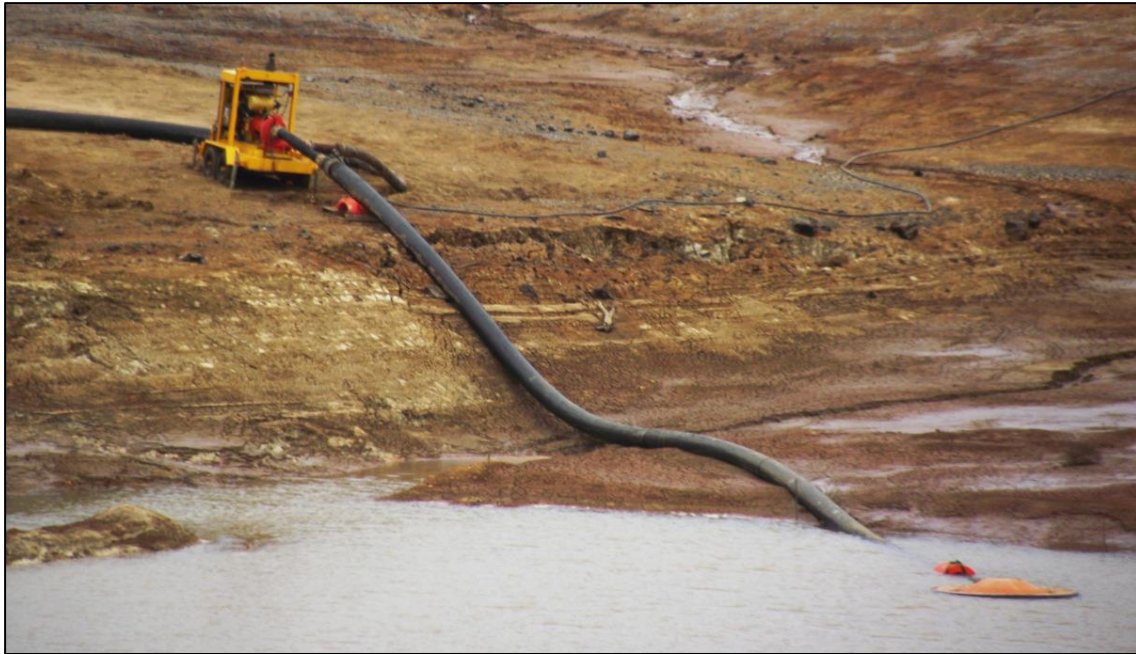
FIGURE 14-2: TURRET SYSTEM POSITIONED IN THE SUPERNATANT WATER CONNECTED TO AN EXTERNAL PUMP
