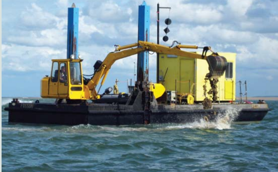
Back hoe dredger at work
