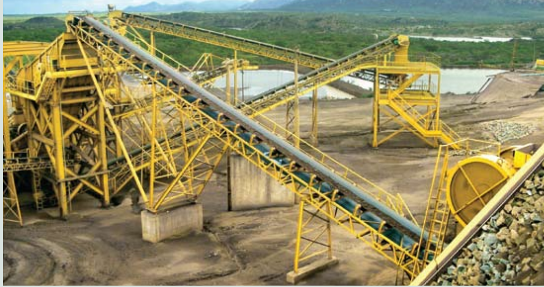
The Mina do Bonito plant
